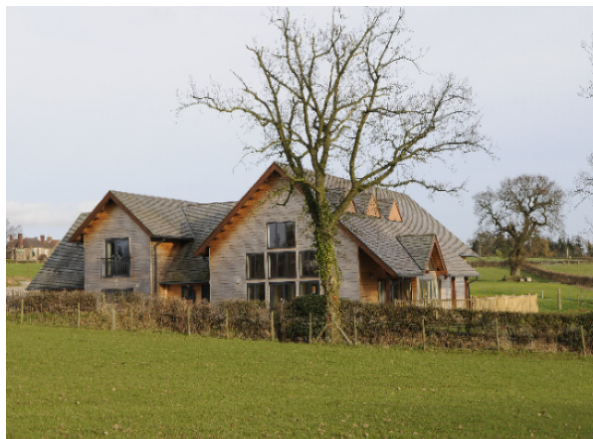
Rock village hall external view
