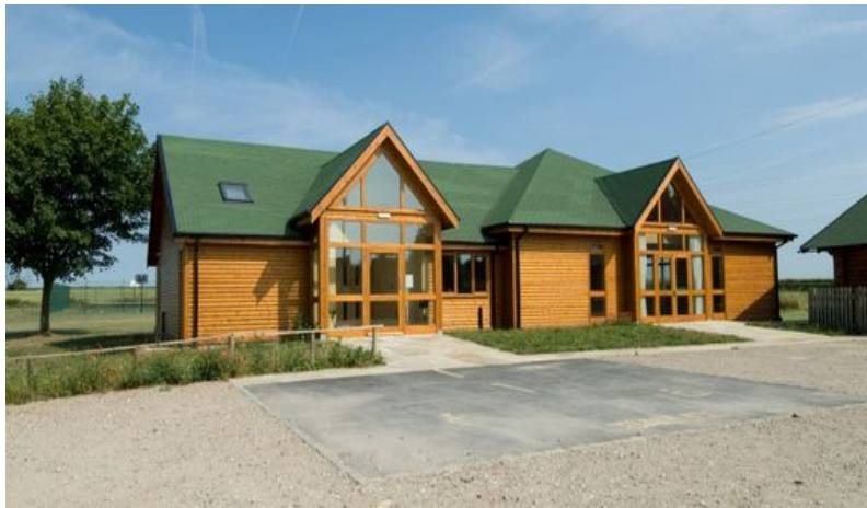
Little Milton external view
