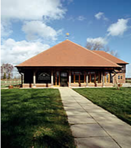
Carpenter Oak Building
